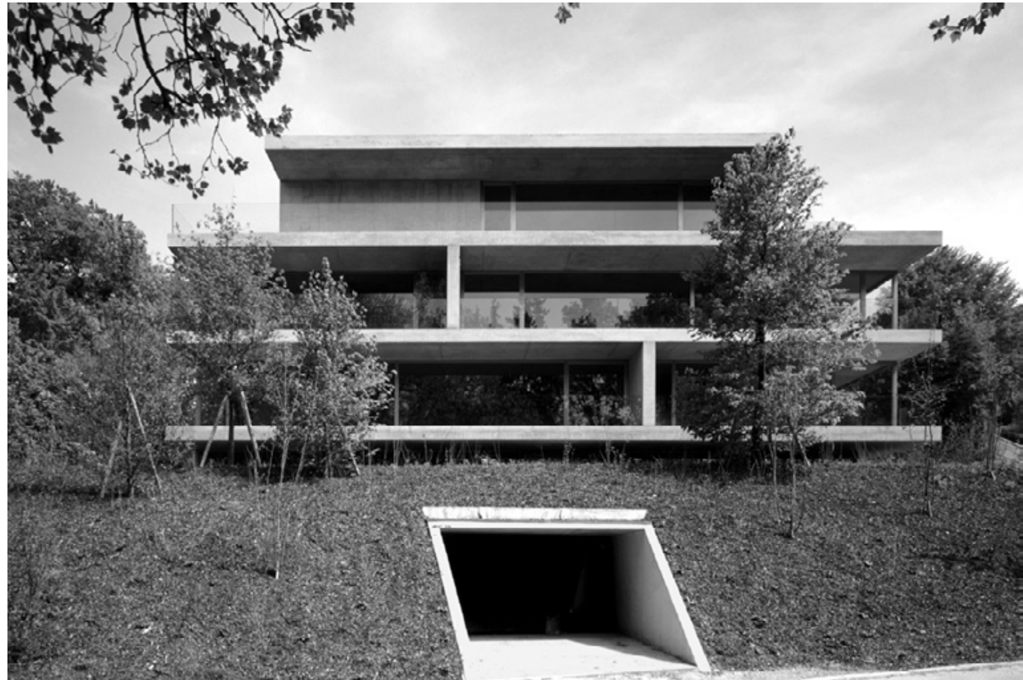
Multiple dwelling Forsterstrasse, Zurich, 2003, Arch.: Christian Kerez, Ing.: Joseph Schwartz
