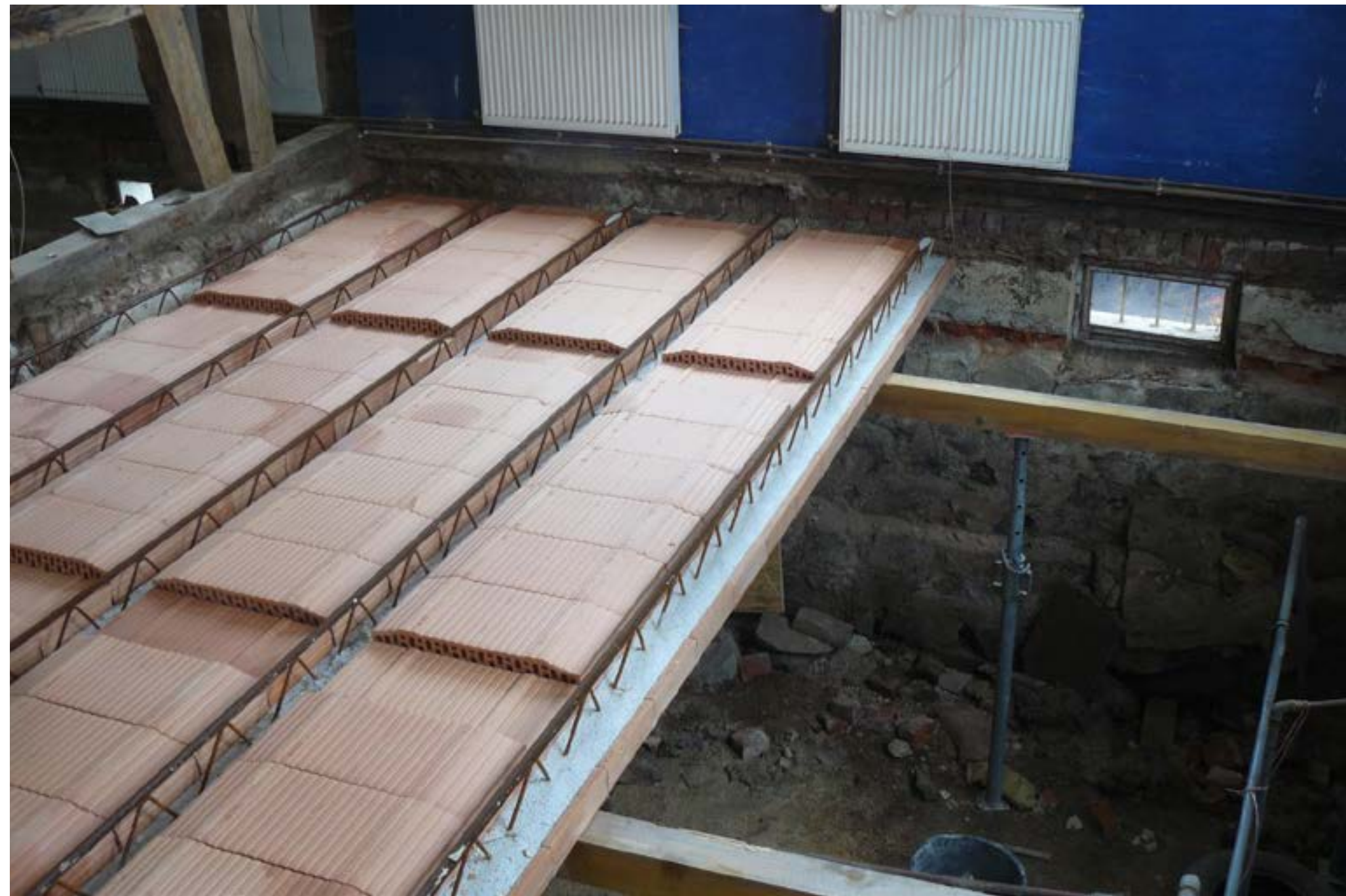
Hollow-gauged brick floor
