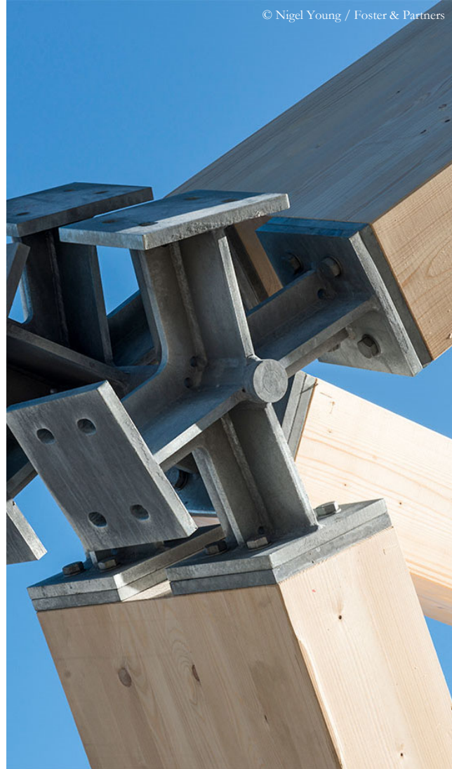
VERSCHRAUBT SCREWED (Canary Wharf Station, London)
