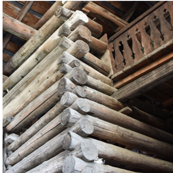
KERBE NOTCH (Singular wall)
