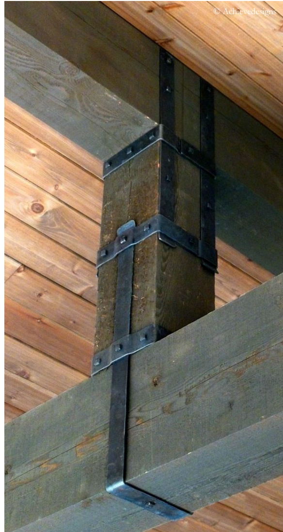
GEBOLZT BOLTED (OWT Timber Bolts)
