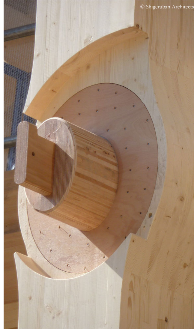
DREHGELENK SWIVEL JOINT (Tamedia Office Building, Zürich)
