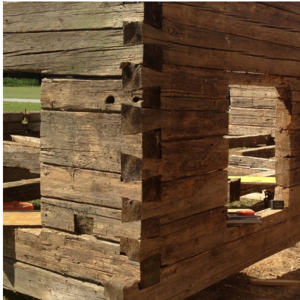
SCHWALBENSCHWANZ DOVETAIL (Singular)
