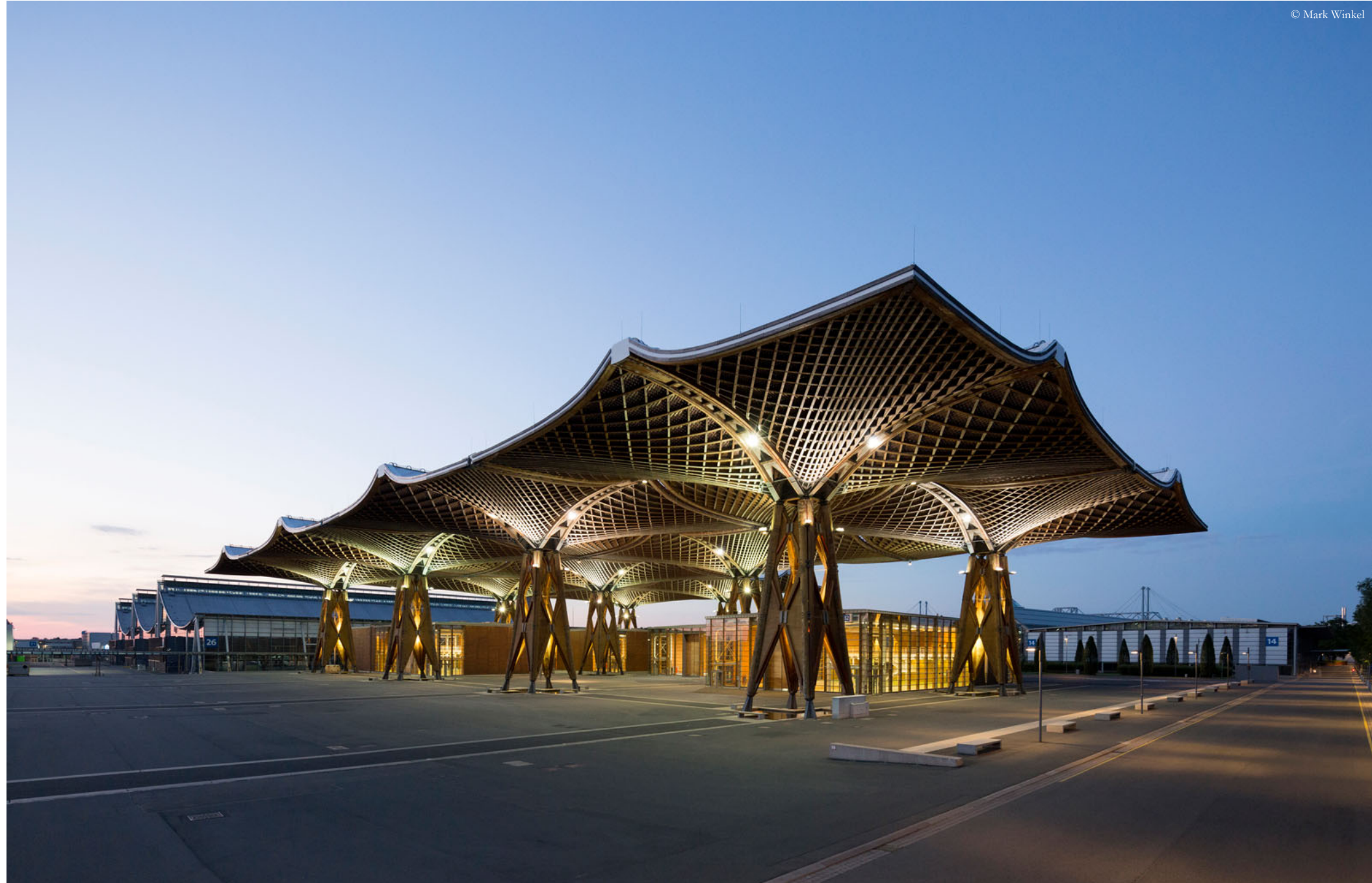
Expo Dach, Hanover, 2000, arch. Herzog & Partner, eng. IEZ Natterer GmbH
