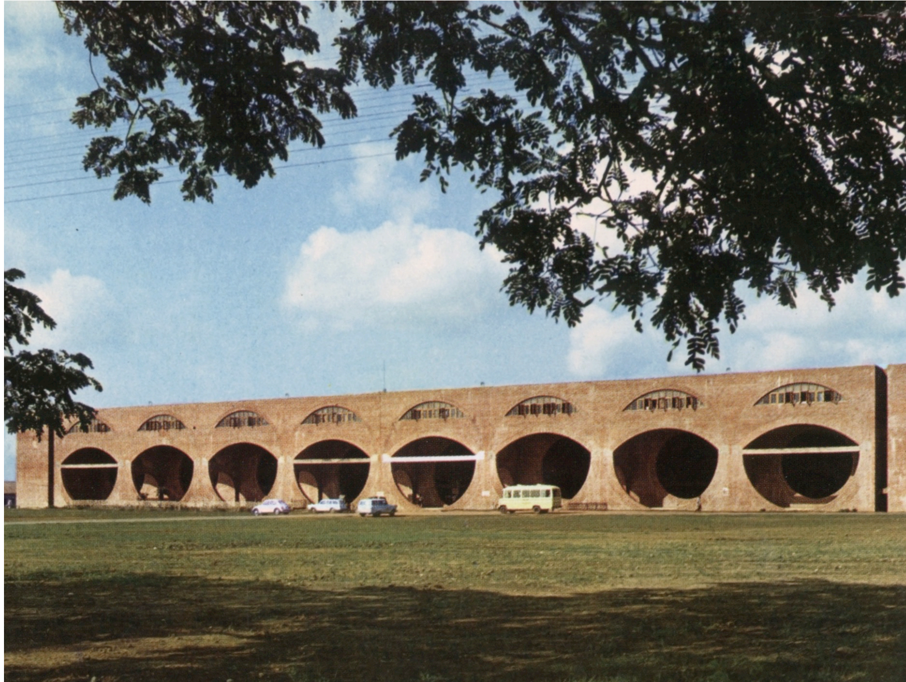
Dilatationsfuge, Louis Kahn, Ayub National Hospital, Dhaka, 1965-1969
