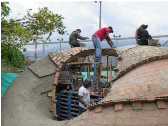
Figure 10: a) The retaining "fins" can be noticed, and b) layout of bricks forming the "fins".
