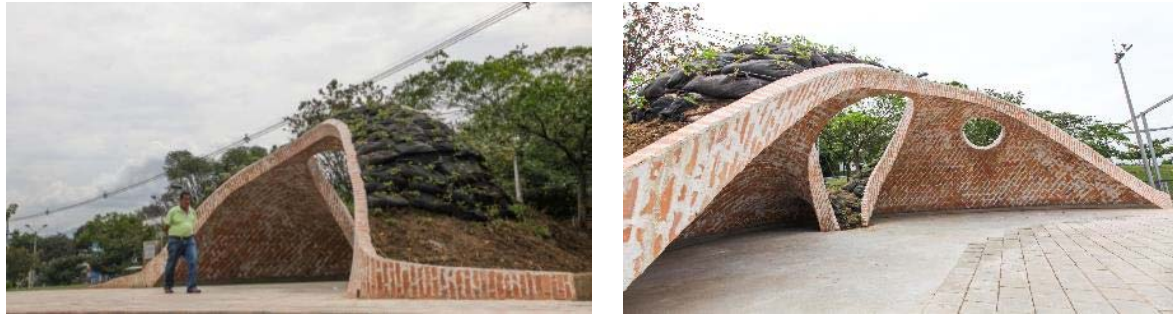
Figure 11: Fotos of the finished construction. © Sergio González
