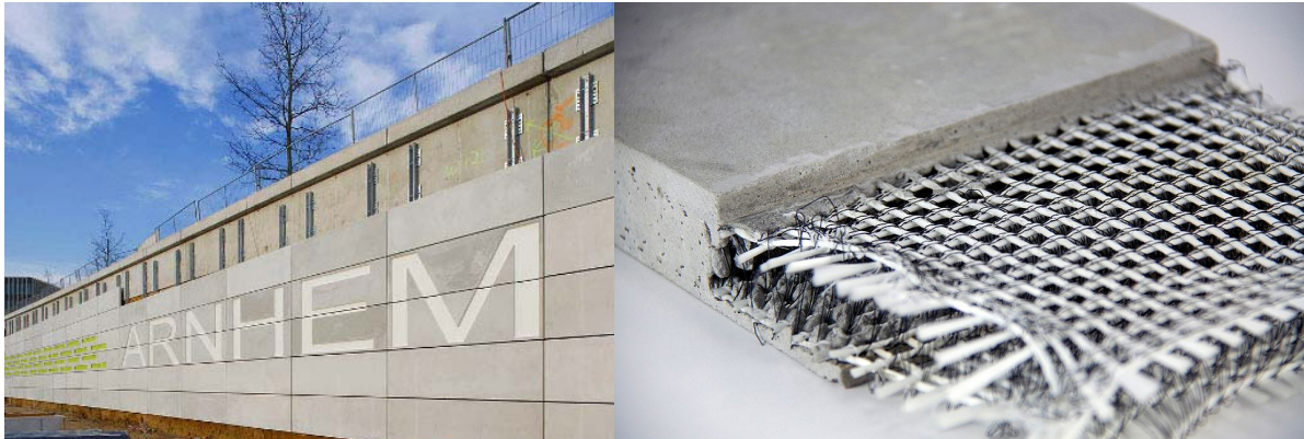
Figure 2: Textile reinforcement, betoShell ® used for facade at Arnhem Central Station (image: Robert Mehl, Hering[6])
