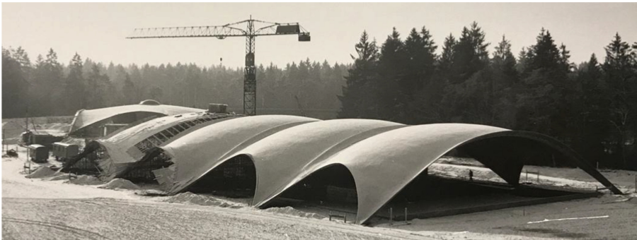
Fig. 1. Isler's "HIB" shells during construction, Heimberg, 1978 (217-0384, gta Archives, ETH Zurich).
