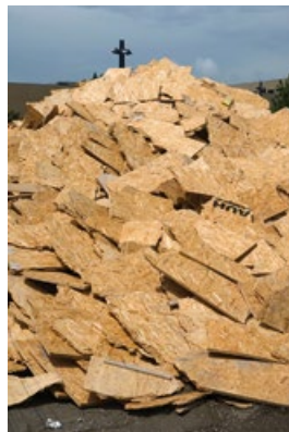
designtoproduction, Destroyed formwork of SANAA's Rolex Learning Center, Ecole Polytechnique Fédérale de Lausanne (EPFL), Switzerland, 2009
