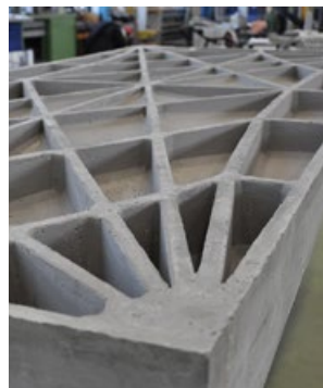
above: The structural system of the HiLo floor is a thin funicular vault made of unreinforced concrete, stiffened by a system of fins on its extrados and supported at its four corners by the primary structural frame. Connected by tension ties to absorb the horizontal thrusts of the funicular shell, the solution results in a thickness of only 2 centimetres (0.8 inches) for both vault and fins.
