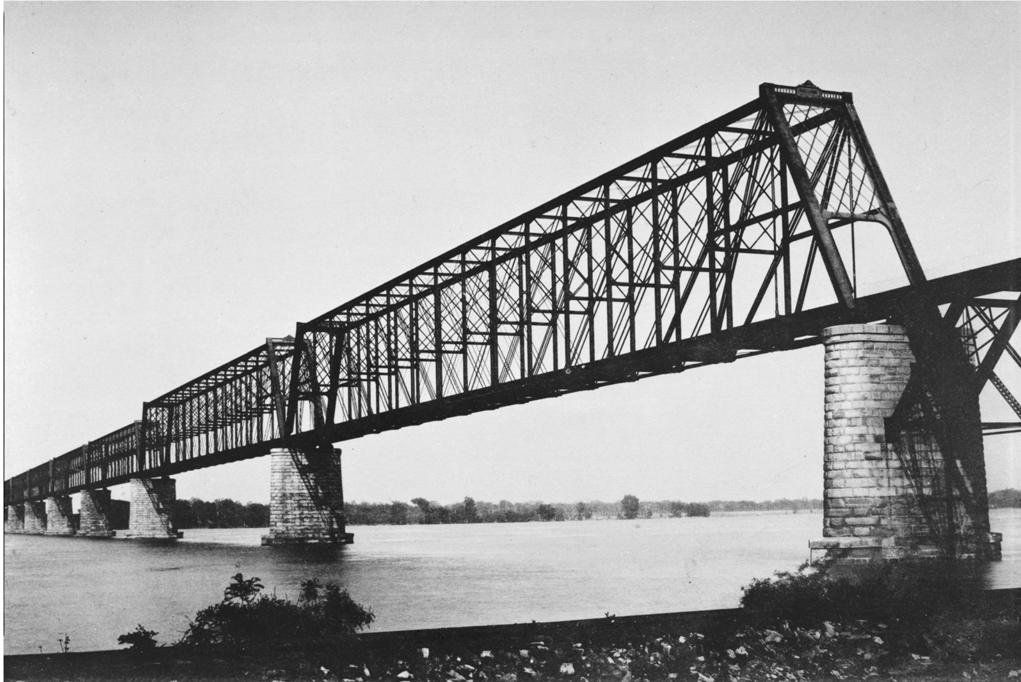
Squire Whipple, Cairo Rail Bridge, Illinois, USA, 1899
