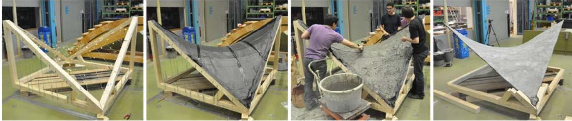
Figure 1: Sequence of construction of the first prototype, and the finished shell.
