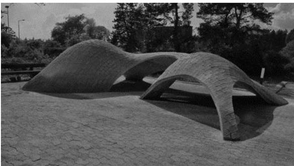
Fig. 5: Prototype of freeform unreinforced masonry vault at ETH Zurich. [11]
