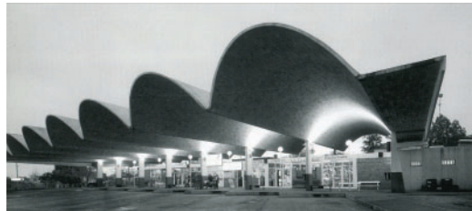
Figure 4. Salto municipal bus terminal, Uruguay. Eladio Dieste, 1973–74 (Anderson 2004).
