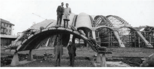
Figure 11. Load test of an “undulating voussoir”, Oviedo’s Sports Palace (1961–1975). Ildefonso Sánchez del Río (Cassinello 2011).
